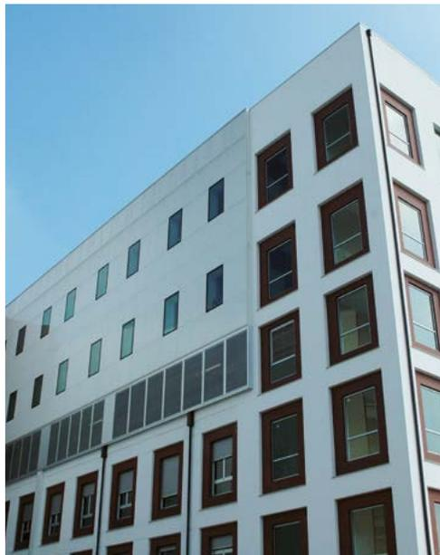
Rivestimento parete isolante in Alucobond / Curtain wall
